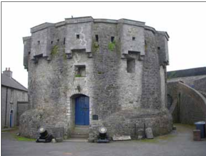
Athlone Castle. The central Keep, a largely 19th century rebuilding using the 13th century battered base of the earlier tower as a plinth.
