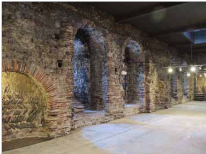
Western outer wall showing inserted fireplace and window embrasures at first floor level.
