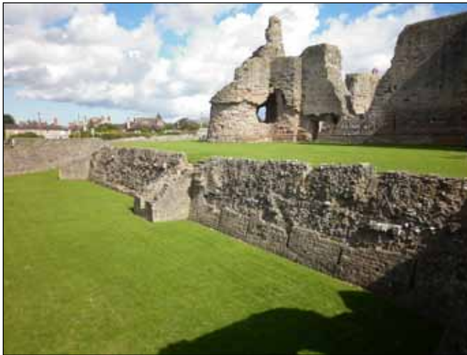
Showing the two sections that may have had a gallery along the base of the outer ward wall.
