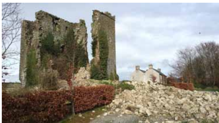
Coolbanagher Castle, Laois, after the storm of 14 February 2014. The fallen masonry of the eastern facade lies below.
