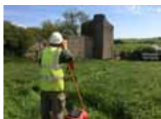
Gleaston castle. Survey underway.
