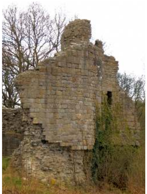
Caergwrlle Castle - from the north. East wall with pentagonal buttress to the left; probable site of entry gate centre and north tower to the right (and below right). North tower D-shaped but rather segmental externally. East tower foundations only, but segmental externally and polygonal internally. South tower probably the keep, fully cylindrical, but perhaps never completed. The castle appears to be unfinished. Plan © Cambrian Archaeological Association. Reproduced with thanks.
