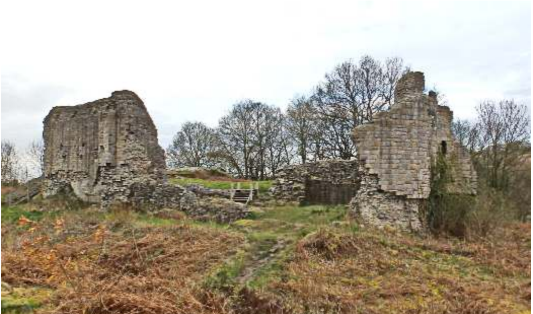
Caergwrlle Castle - from the north. East wall with pentagonal buttress to the left; probable site of entry gate centre and north tower to the right (and below right). North tower D-shaped but rather segmental externally. East tower foundations only, but segmental externally and polygonal internally. South tower probably the keep, fully cylindrical, but perhaps never completed. The castle appears to be unfinished. Plan © Cambrian Archaeological Association. Reproduced with thanks.
