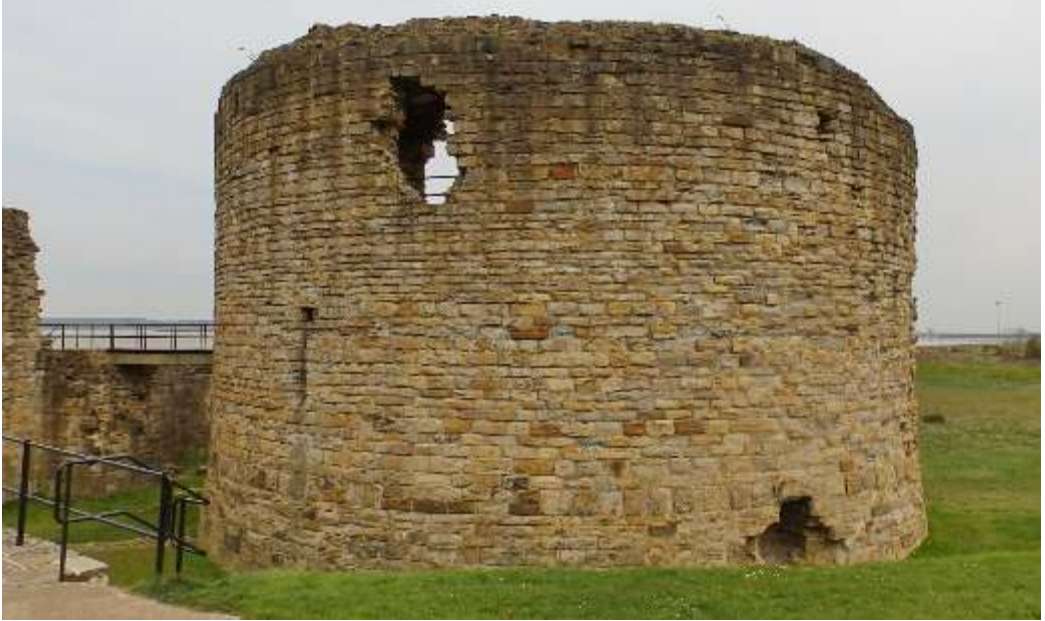
ABOVE: Fig. 7. Flint, the Great Tower, from the SW. For affinities and possible origins see John Goodall, 'The English Castle', 2011, pp 213-4. Some suggest that the Tour de Constance at Aigues Mortes 'virtually complete by 1266' (Bothamley in Arch J. 73) might be a model. Note band of large square ashlar above the plinth.
