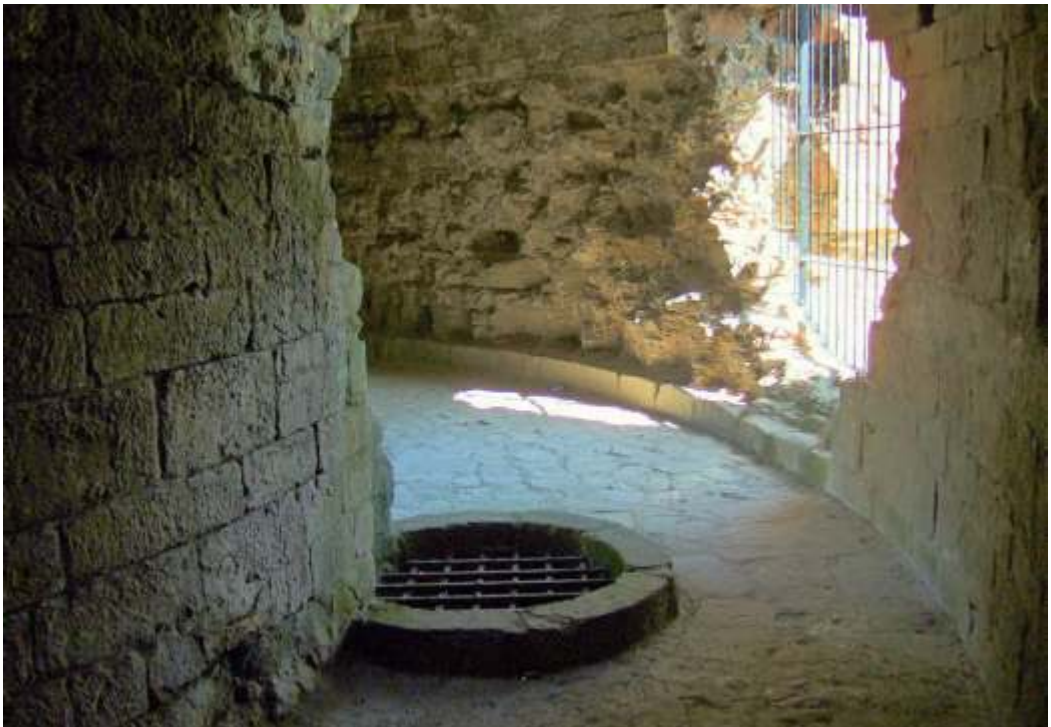
BELOW: Fig. 11. The stone-vaulted gallery running around the basement of the Great Tower. It is narrowed at one point by the well, situated near the enlarged loop in the south (seen above). The vaulting pattern within the embrasure suggests, possibly, that this opening accommodated a postern.
