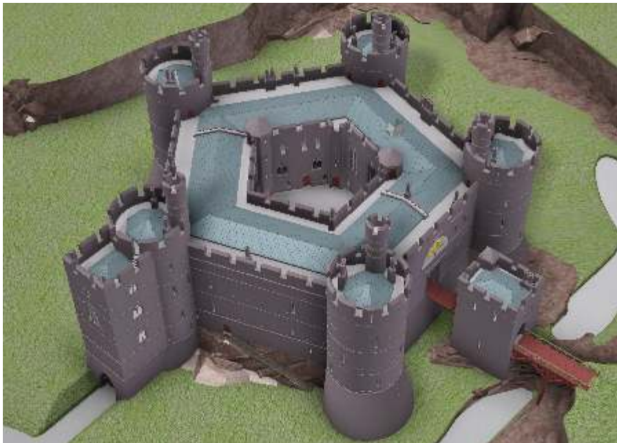
BELOW: Fig. 13. High level view of the model from the north east showing the three spiral staircases in the courtyard, only two of them complete to wall-walk level
