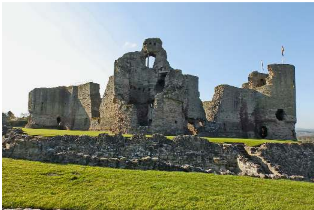
BELOW: Fig. 4. Rhuddlan Castle from the north. North Tower, centre, West Gatehouse, right; turreted steps down to the moat foreground. These series of steps (4, N & E sides were probably walled and roofed for protection).
