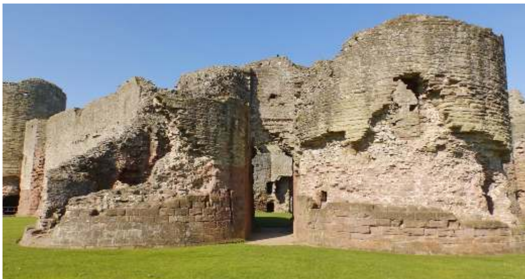
ABOVE: Fig. 5. The East Gate. Similar to the West Gate. Four ground floor arrow loops per tower.
