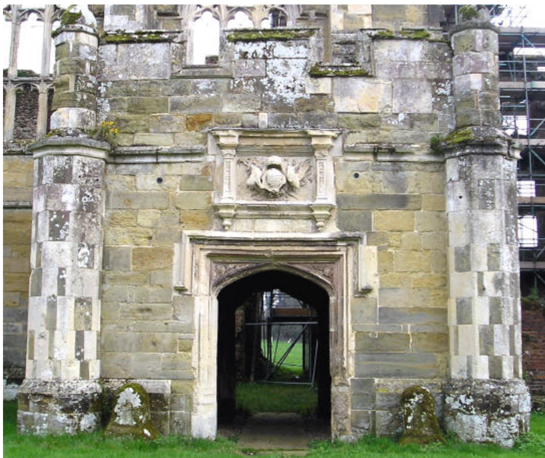
Fig 9 Cowdray House. Late 1530's entrance porch to the Great Hall, added by Sir William Fitzwilliam, giving access to the screens passage, with the hall to the left. The Great Hall has three perpendicular windows, high up, each of three lights with cusped heads and a transom. The motif of the alternate white and dark- polychrome - ashlar is carried forward from the gatehouse into the mini turrets
