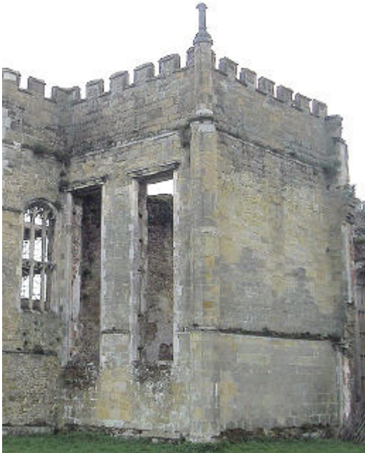
Fig 12 Cowdray House. The stairwell block adjacent to the Chapel that houses the stairway to the first floor apartments. There had been long windows in the north wall (now blank) blocked in the early eighteenth century to accommodate the Pellegrini paintings.
