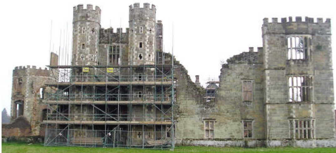
Fig 3 Cowdray House. The west, gatehouse facade. Gatehouse circa 1535-40 with alternating nominal gun loops and decorative arrow slits. The canted bay windows in the NW and SW corner towers were probably later. The Heritage Lottery Fund have recently agreed to a £2.7 million campaign of conservation and the consolidation of the Gatehouse is the first phase of this work.
