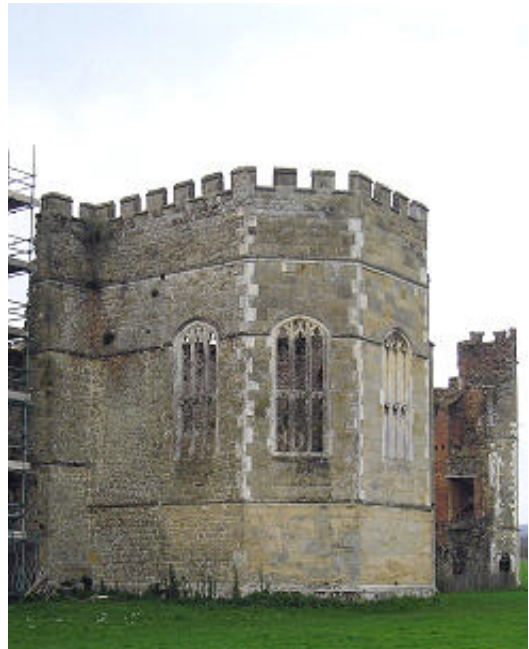
Fig 13 Cowdray House. The Chapel - 1520-30. The three-sided apse. The chapel's position behind the Great Hall is similar to the location of the chapel at Thornbury. The crenellations are a later addition, circa 1535.
