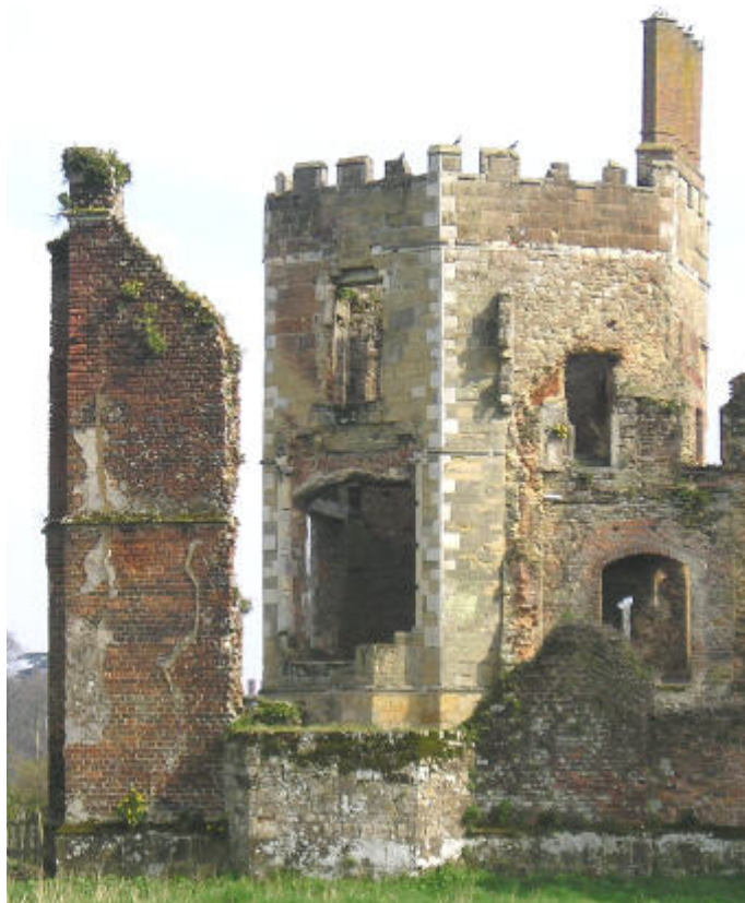
Fig 24. Cowdray House. The hexagonal residential tower in the north-east corner, with its fashionable pattern of interlocking brown and white quoins. The huge bay window is probably a later Elizabethan enlargement.
