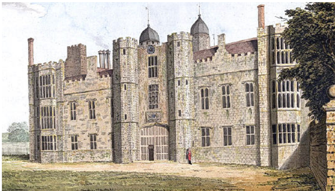
Fig 1. Cowdray House - The west, entrance façade, completed in its entirety by 1545. The Gatehouse was constructed in the late 1530's, of rubble faced with ashlar with white stone quoins. It is of three storeys but has lost its floors and roof. From a watercolour of the 1780's by S H Grimm. BL Shelfmark: Additional MS 5675, f. 11 (no. 17). All the Grimm paintings in this article are reproduced by kind permission of the British Library.
