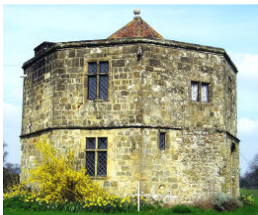
Fig 4 Cowdray, The Conduit House. All the rooms are triangular as they radiate from a central pillar. It is now called the Round Tower and used to be the home of the resident custodian.
